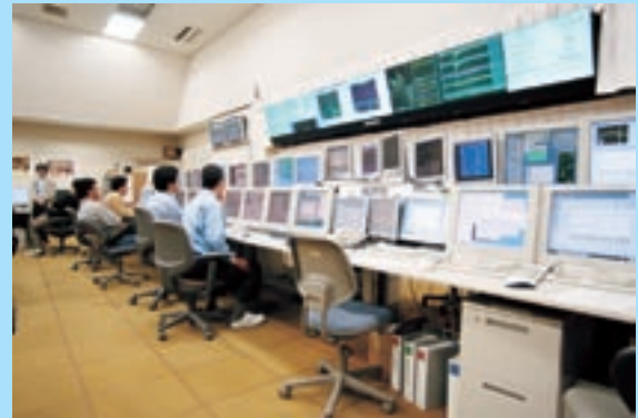
Control room: Accelerator scientists control KEKB's many pieces of equipment from the central control room. Many monitors are lined up to display the current status of the accelerator. The central control room also controls equipment at sub-control rooms located around the ring.
